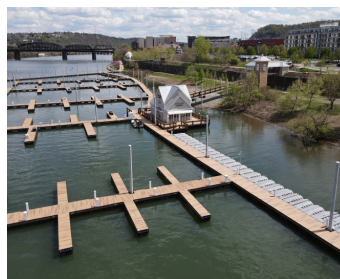
New floating dock with finger piers
