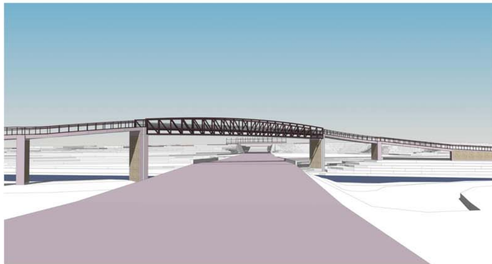
ROOSEVELT WESTBOUND VIEW (RT. 59 BRIDGE IN DISTANCE)
